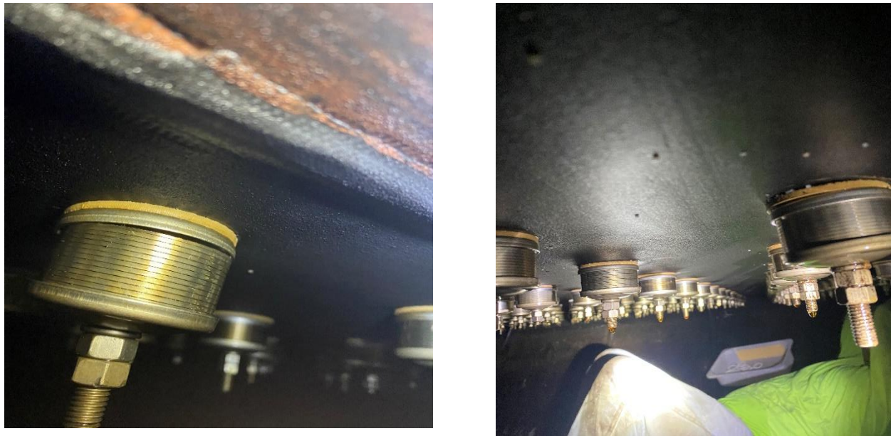
Figure 6: Examples of Misaligned Nozzles
