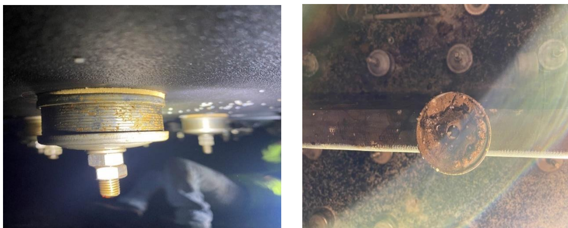
Figure 8: Nozzle Buildup – External (left) and Internal (right)
